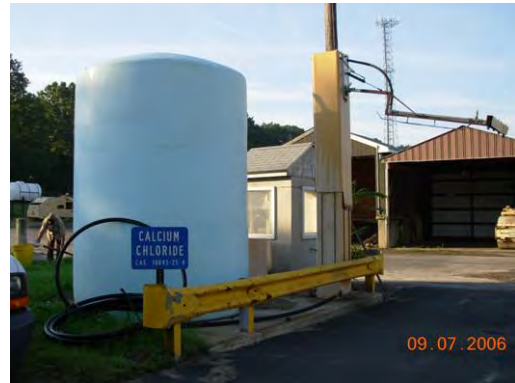
Figure 38. Overhead Pre-Wet Spray System
